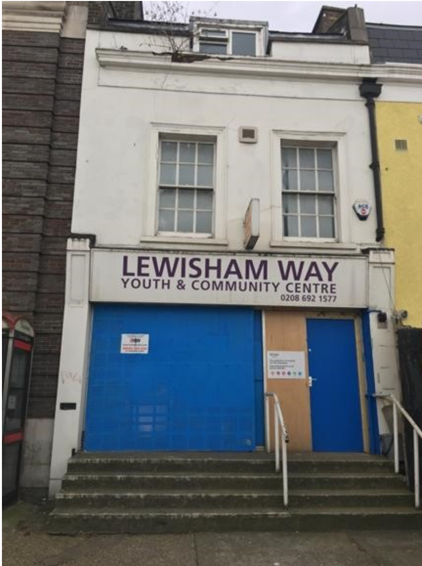
Image description: Lewisham Way Community Centre following the Youth and Community Centre's vacation – note the temporary security screens, signs confirming the presence of live in property guardians and alterations made to frontage to accommodate the presence of live in property guardians.
